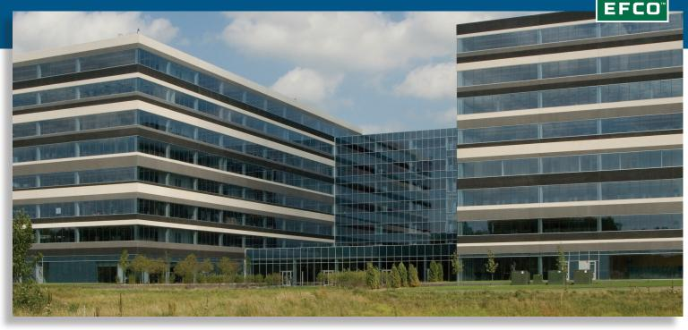
Outside Glazed • Inside Glazed • 2 or 4-sided Structural Silicone Glazed The 5500 2-1/4" curtain wall system is designed to meet the most demanding performance specifications. System 5500 utilizes the E-Strut thermal isolator, providing outstanding thermal properties and a total composite shape for enhanced structural performance. System 5500 offers dual finish capability to meet any design finish specification.
